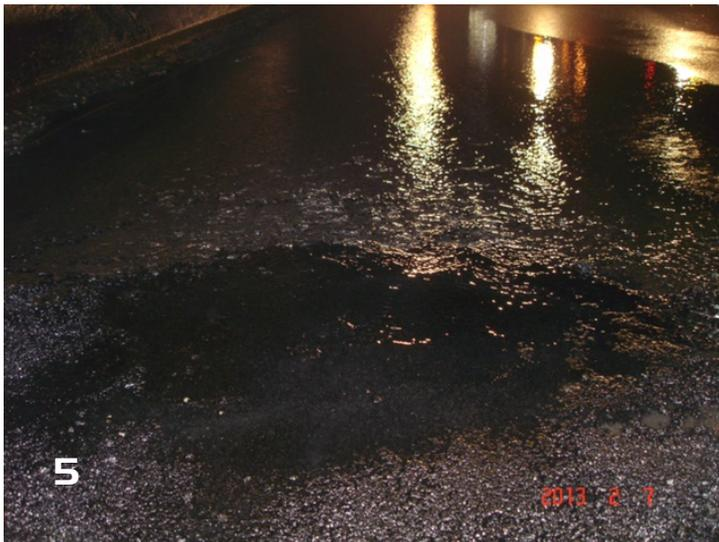
This was a pothole that was approx. 10" deep, down to the concrete below. Massive amount of sea water running out of it right in the wheel path of the right lane. Filled it with Aquaphalt to safe up the lane until we did the joint repair in this location. Aquaphalt stayed in place until the repair was performed.
