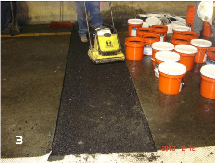
We placed the Aquaphalt in 2 lifts to make sure it didn't settle too much with the heavy traffic volume on Interstate 664. In one instance when we came in the next night, one of the patches did settle about  $\frac{3}{4}$ " so I tried putting a skim patch on top of what we did the night before doubting that it would adhere and stay in place. Not only did it stay in place there was water still seeping out of this patch. This was approximately 3 years ago and it is still in place.
